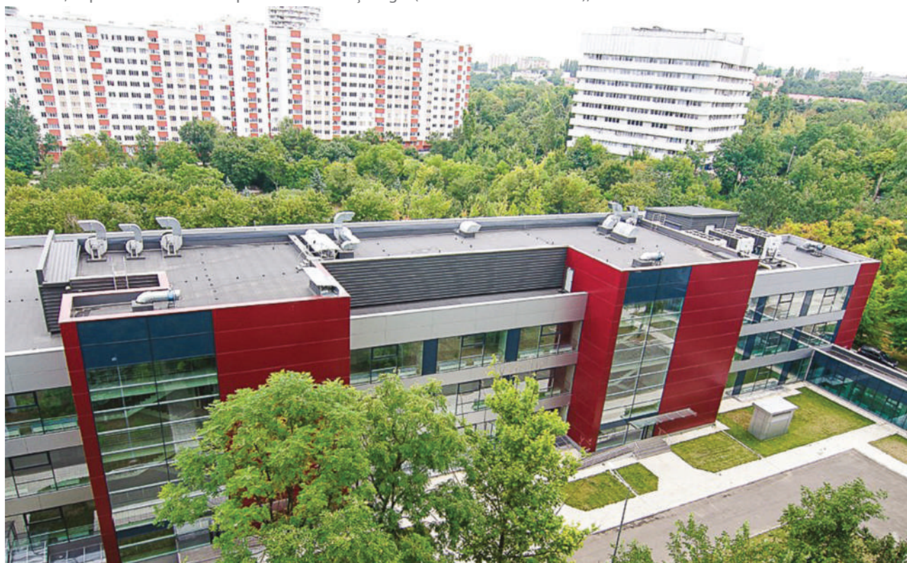
▼ Blocul chirurgical, Spitalul Clinic Republican „Timofei Moșneaga” (vedere de la etajul al 10-lea), vara 2017 / Surgical Department, Republican Clinical Hospital „Timofei Moșneaga” (view from the 10 th floor), summer 2017
